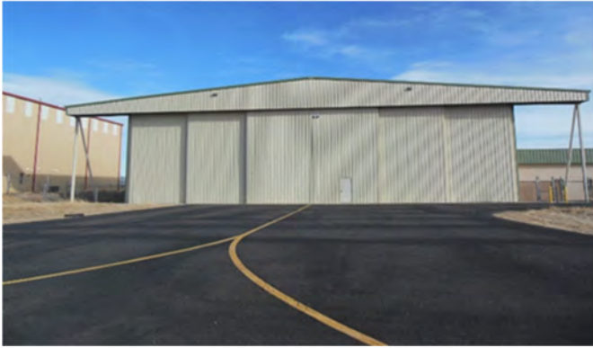
Conventional Hangar (Exhibit 1J – #5)
