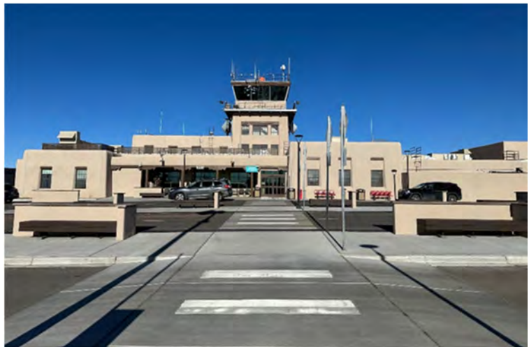
SAF Terminal Building (Front)
